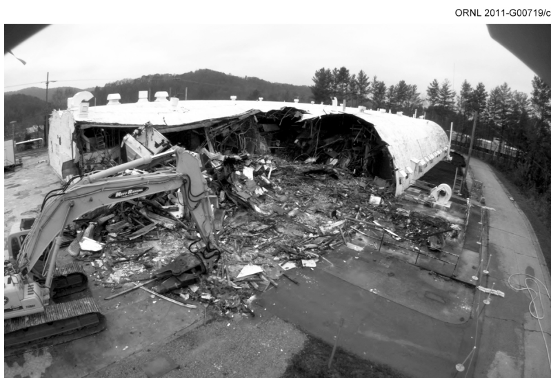
Fig. 5.4. Demolition activities at Building 2000.
